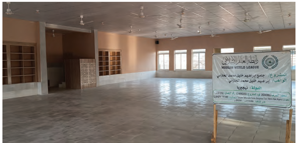
Al-Hazmi Mosque through the construction phase
