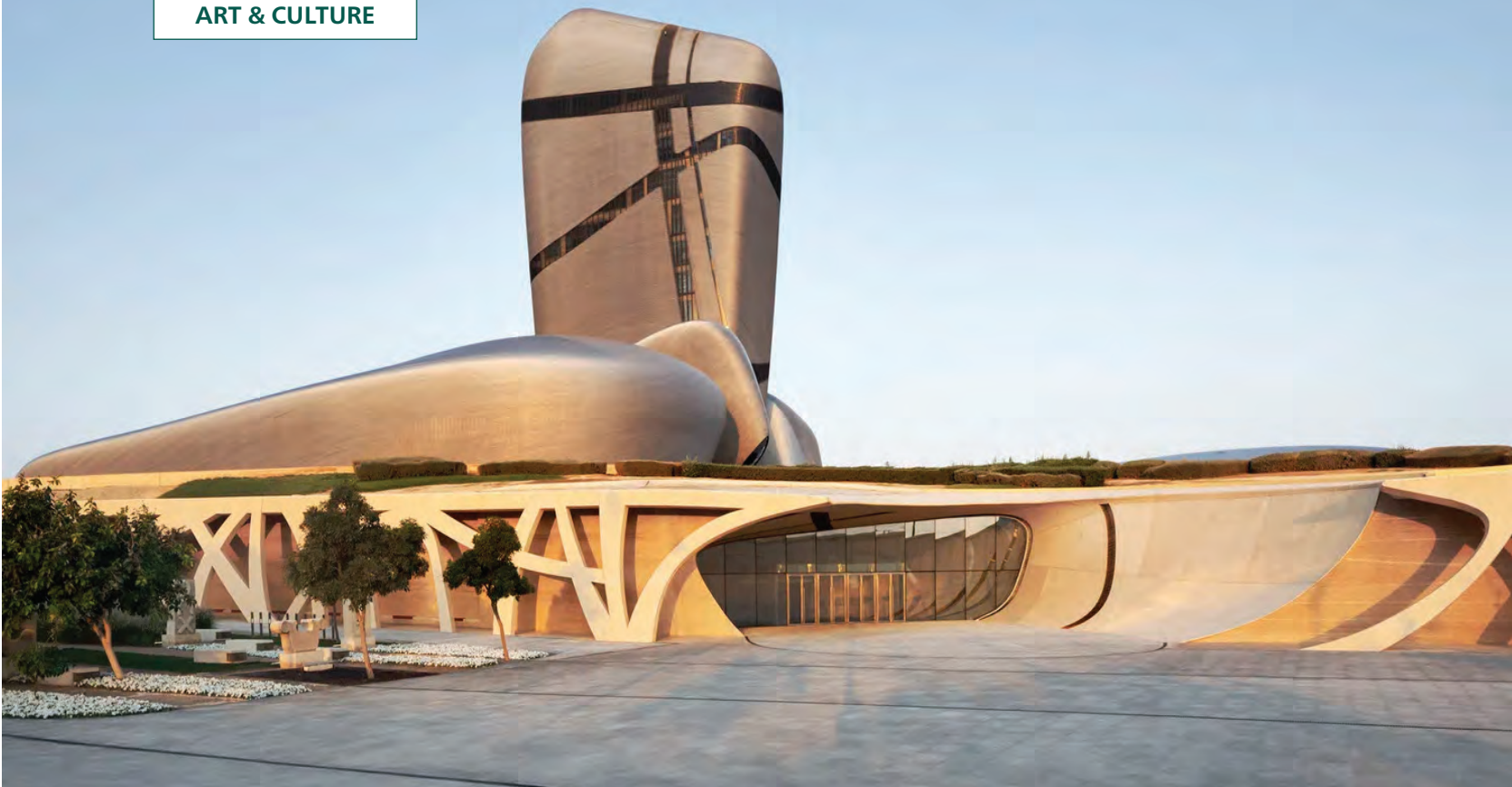
King Abdulaziz Center for World Culture (Ithra), Dhahran, Saudi Arabia — contemporary architecture inspired by regional landscapes and heritage
