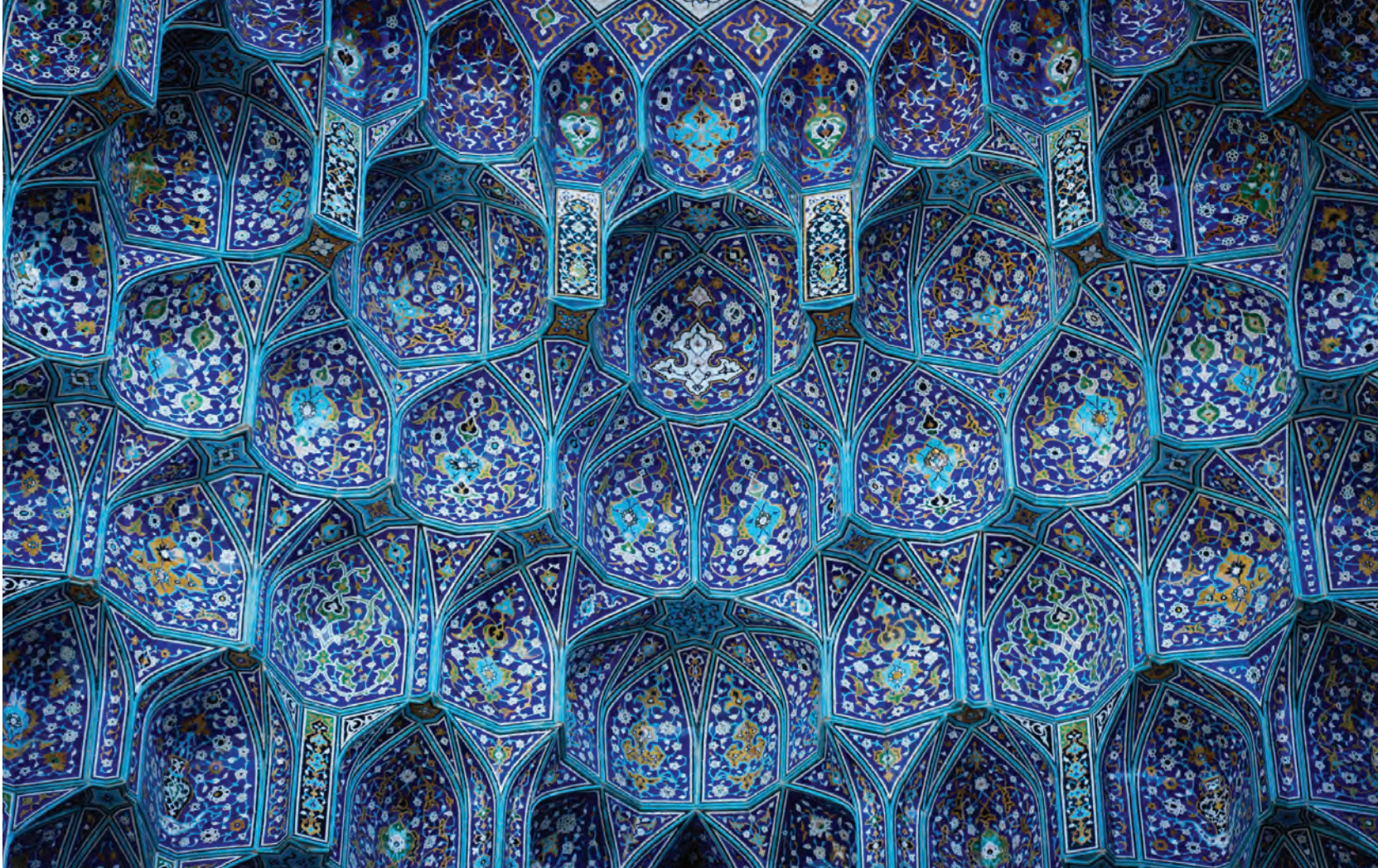
Muqarnas vault with blue tilework, Persia with geometric and floral patterns in glazed ceramic
